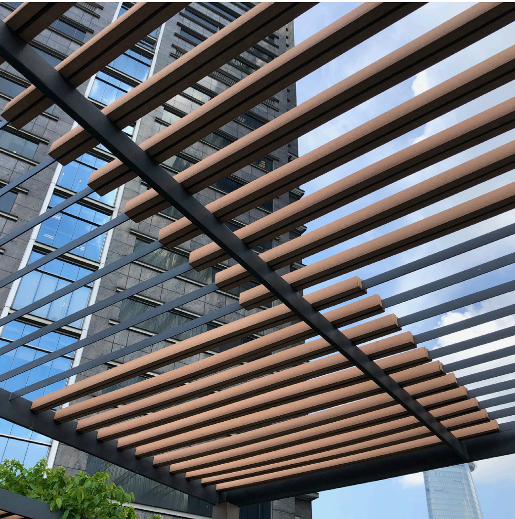
Integrated timber and steel pergola providing shade and amenity
